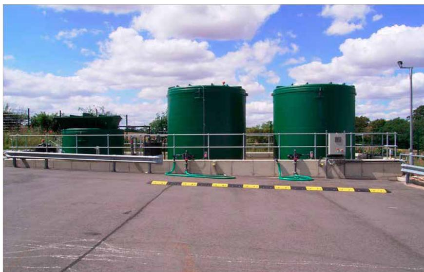
**Vertical storage tanks (the large tanks shown are 50, 000 litre capacity)**
